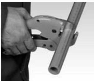
Cutting of the pipe
