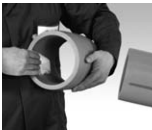
Clean the inner surface of the electrofusion socket
