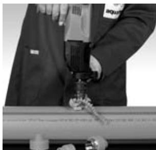
Drilling through the pipe wall
