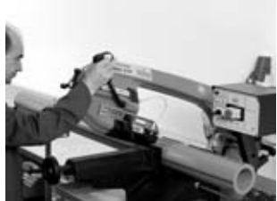
Before welding, the 160-355 mm pipes are cut into the required lengths
