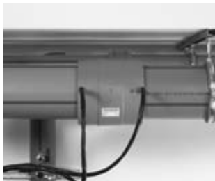
Adjust the socket diameter on the welding device. Start and control welding process. Keep the cooling time. Finished!
