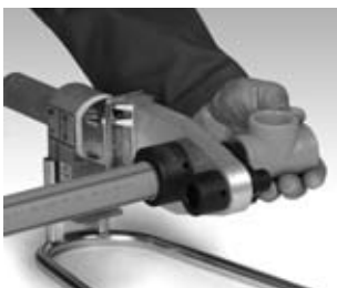
Heating-up of pipe and fitting
