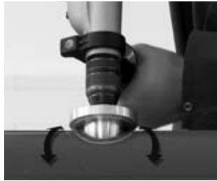
Removal of the oxygen barrier layer from the climatherm OT-pipe
