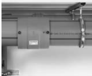
Push the second pipe - also peeled and cleaned - into the socket
