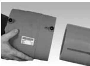
Push the electrofusion socket onto the pipe end
